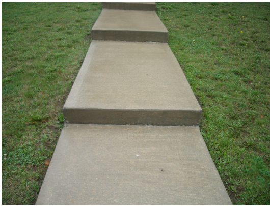
(a) Stairs 1. Found in front of the town homes in Columbia Lake Village. Rise: 7.2 inches, Run: 86.2 inches, Width: 48.5 inches, Overlap: 0.5 inches, Slope: 0.0835, rise + run: 93.4, rise * run: 620.64 , 2*rise + run: 100.6 , Feel: Safe, and full three foot steps on each step
