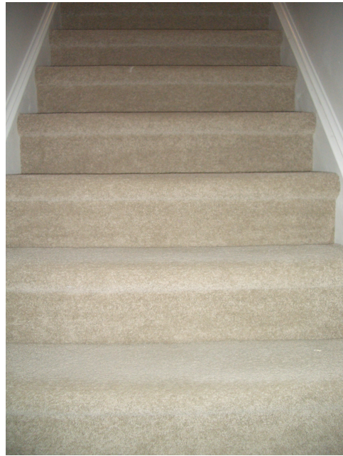
(b) Stairs 2. Found in my friends home. Rise: 7 (inches), Run: 9.5 (inches), Width: 36 (inches), Overlap: 1 (inches), Slope: 0.737, rise + run: 16.5, rise * run: 66.5 , 2*rise + run: 23.5, Feel: Ok going up, step feels a little too small, my foot only just fits the whole step. The overlap affects the decent a little, makes it somewhat uncomfortable.
